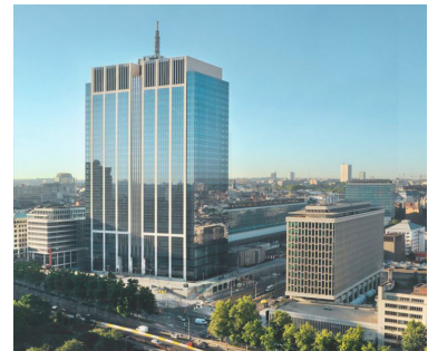
Finance Tower, Brussel Bron: Jaspers-Eyers Architecten
